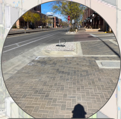
Completed the Mason Street Entrance
