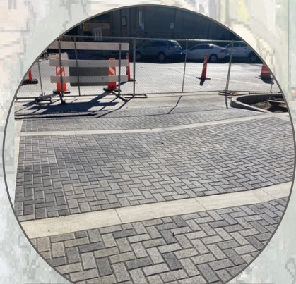
Completed the Olive Street Entrance
