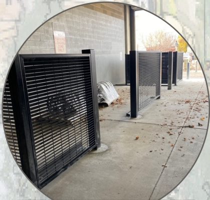
Completion of the trash enclosure installation.
